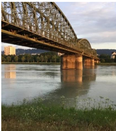
Old railway bridge 1900-2016
